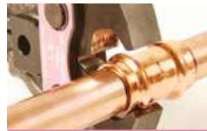
9. Align jaws squarely on the fitting
