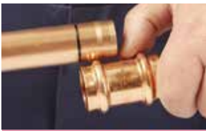
7b. Check the depth mark
